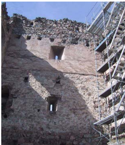
Brienzen, GR, ruined castle Belfort, 13 th century render on the west wall of the „Palas“
