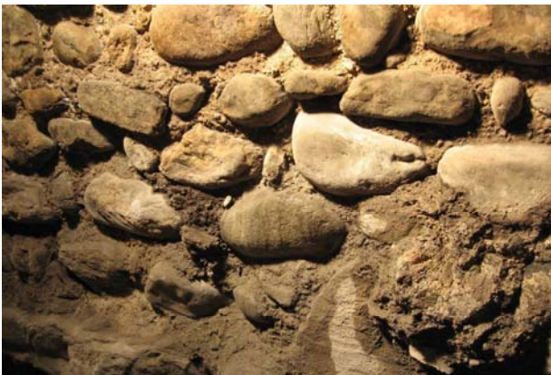
Boulder masonry, around 450 AD, St. Stephan, Chur, GR
