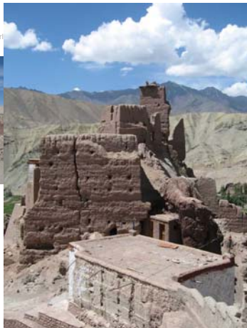
Basgo, Ladakh castle built out of rammed earth (pisé)
