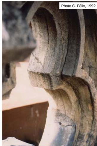
Materials and conservation of built cultural heritage – The weathering of the natural building stones. BR 64
