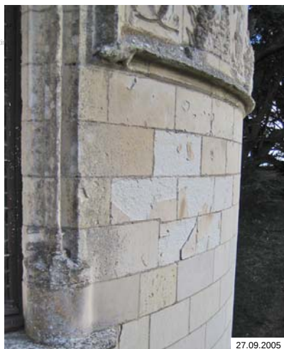
Materials and conservation of built cultural heritage – The weakening of the natural building stones. BP 68
