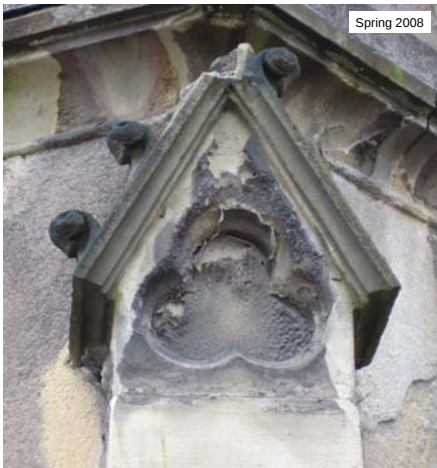
Materials and conservation of built cultural heritage – The weathering of the natural building stones. BP 4/9
