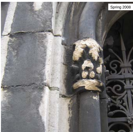
Materials and conservation of built cultural heritage – The weathering of the natural building stones. BP 5/9
