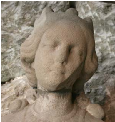
Materials and conservation of built cultural heritage – The weathering of the natural building stones – BP 62
